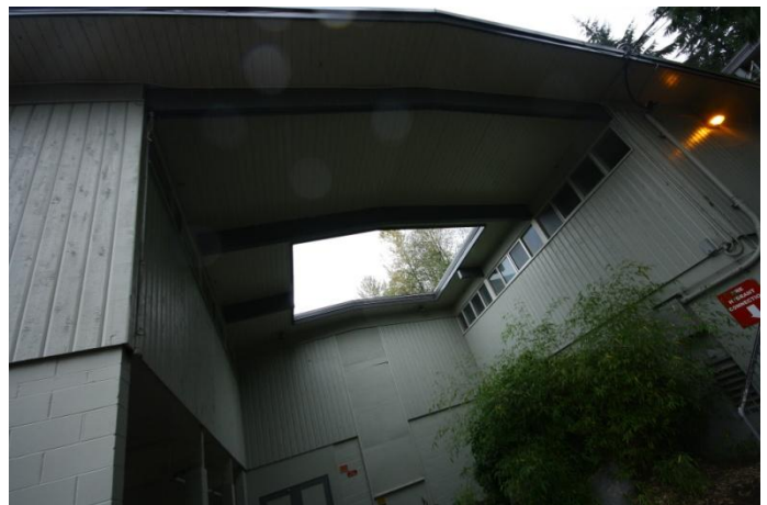
Front entrance roof structure
