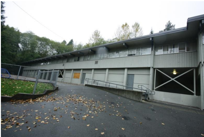
View of South façade
